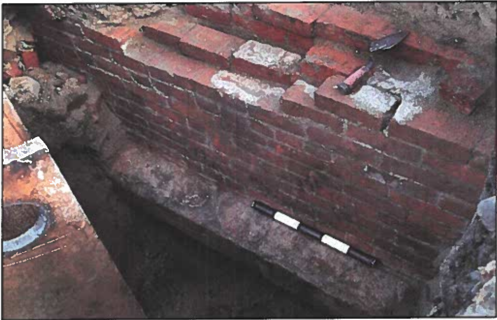
Figure 7. Example of a Buried Brick Foundation
